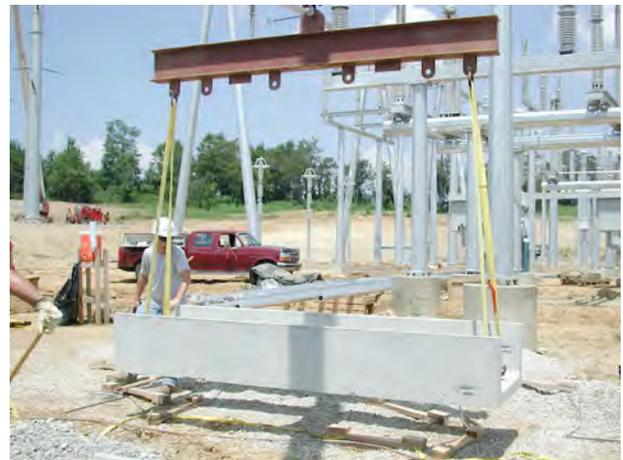
6. Begin the trench base installation at a fixed point such as a building, equipment foundation, manhole etc. then place subsequent base units in sequence per Trenwa's layout drawings. Set the elevation and alignment of the trench bases with an electronic level and a transit. An off set string line can be used to assist in keeping the trench aligned.
